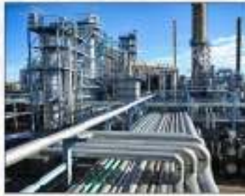
Petrochemical Plant Pipes
