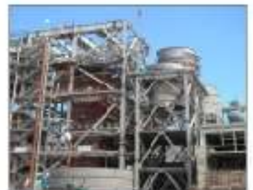
Thermal Power Generation Boilers
