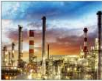
Oil & Gas Plant Pipes
